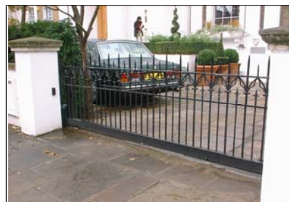
This gate can crush if the closing force is not correctly adjusted and each vertical bar passing the pillar is a potential shearing edge.
